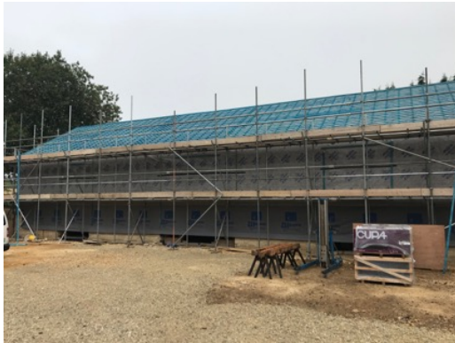
Mickleton Hills under construction
