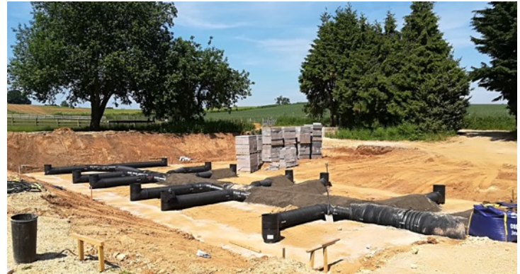
Ductwork installed before concrete foundation laid
